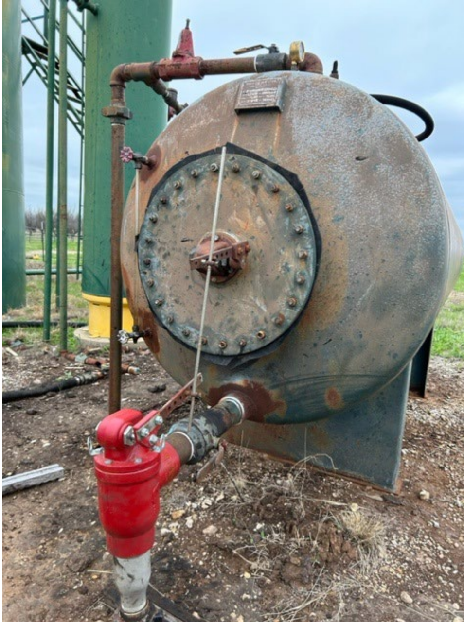
New valves being installed at Piave in anticipation of production. Kalkee 2023
